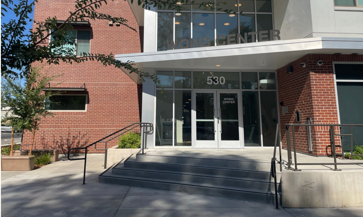
Front of the Building
